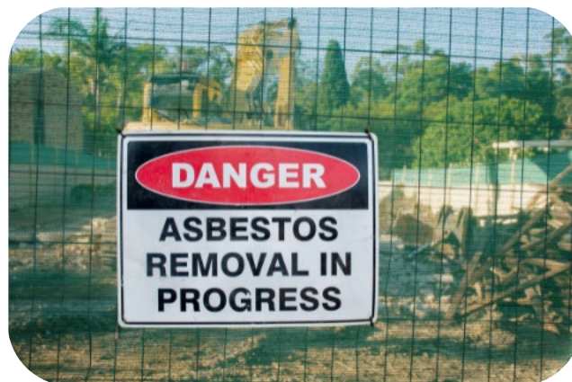
Asbestos fibers typically pose the greatest risk when they are disturbed.
